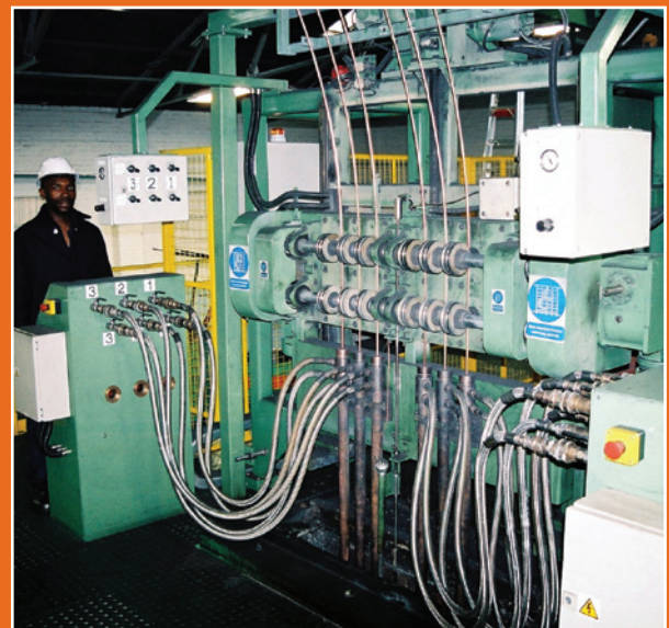
Casting station and strand withdrawal
